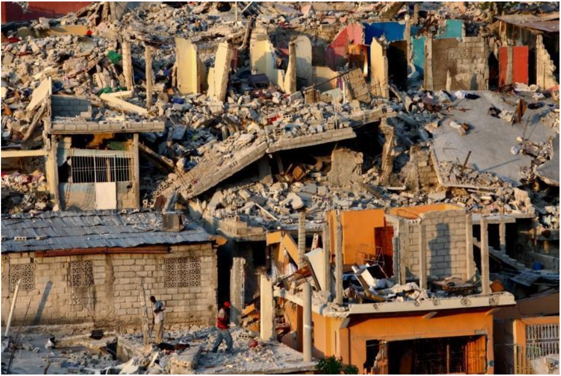
Figure 1 Buildings destroyed in 2010 earthquake in Haiti.
